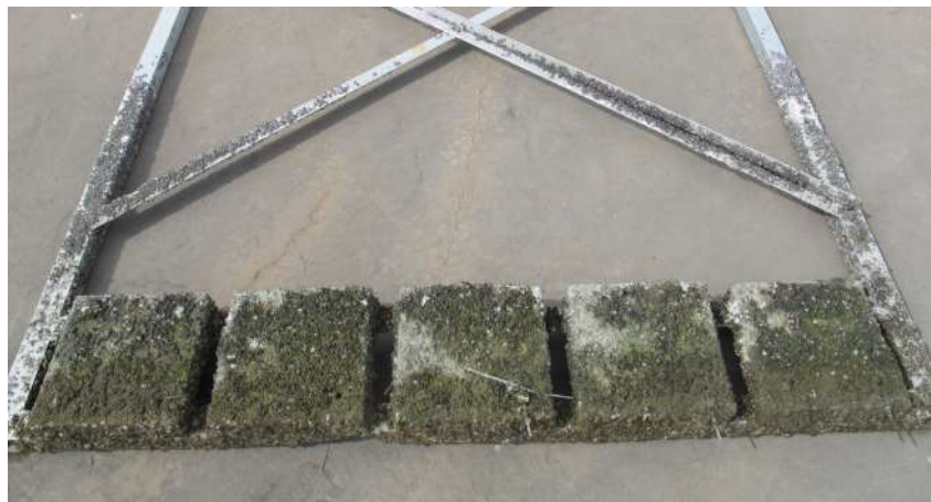
Figure 1. Aluminium framework used to support settlement plates on seawall
